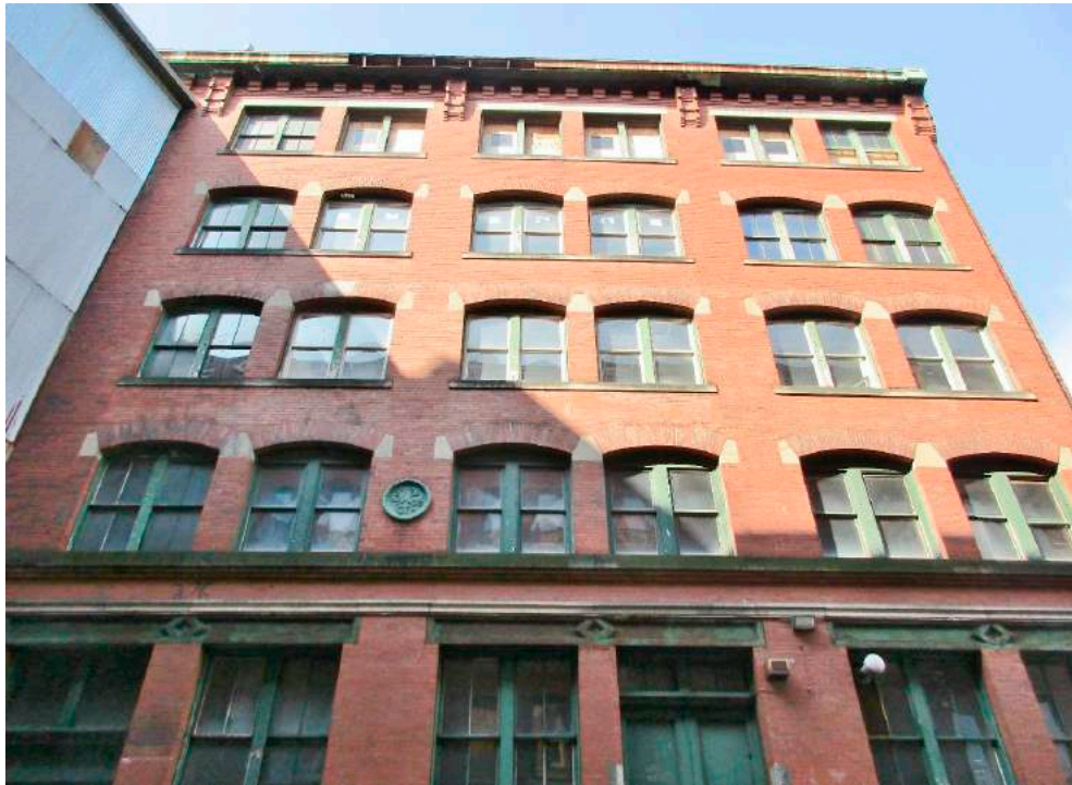
3. View southwest of 6 Necco Court from north side of Necco Court
