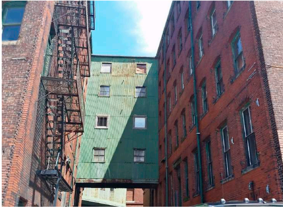
7. View northeast of pedestrian bridge connecting the west elevation of 5 Necco Court and east elevation of 6 Necco Court
