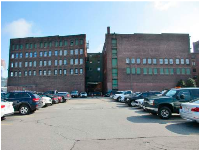
Existing Brick Buildings looking north from site of New Building
