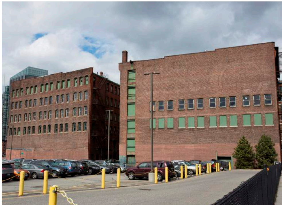
8. View northwest of 5 and 6 Necco Court from west side of Necco Street
