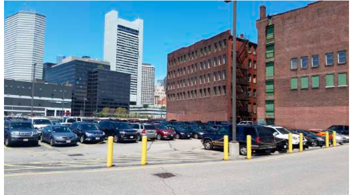
Existing Brick Buildings looking northwest from Necco Street
