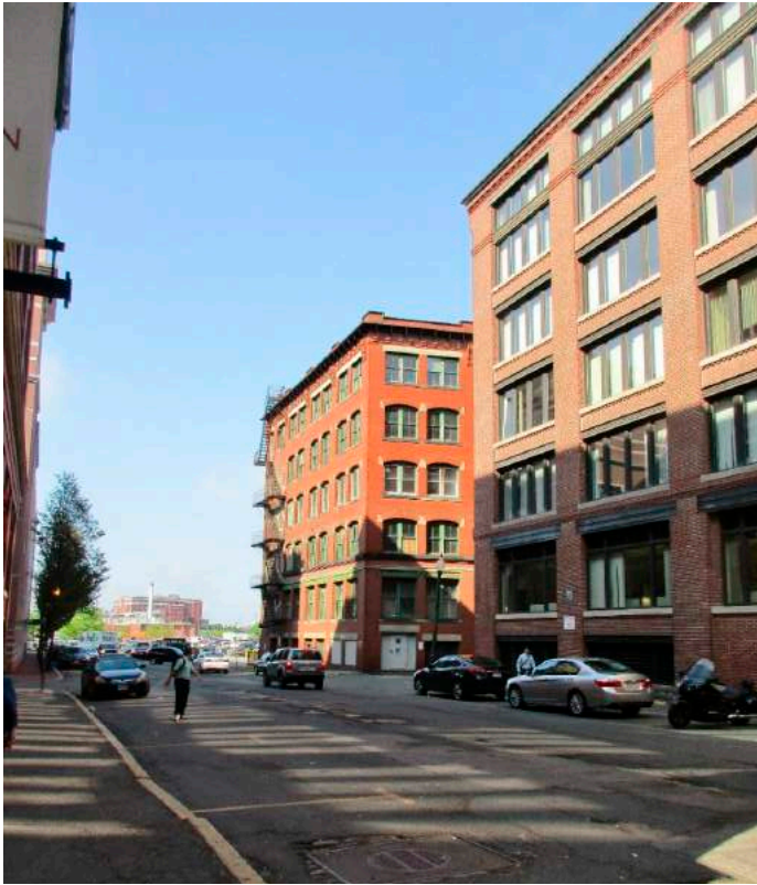
13. View southwest of 5 and 6 Necco Court from intersection of Necco Street and Melcher Street
