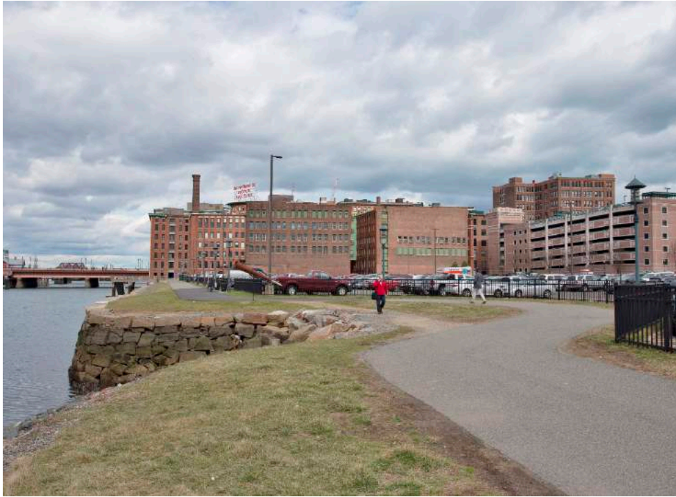
9. View northeast of 5 and 6 Necco Court from east bank of Fort Point Channel
