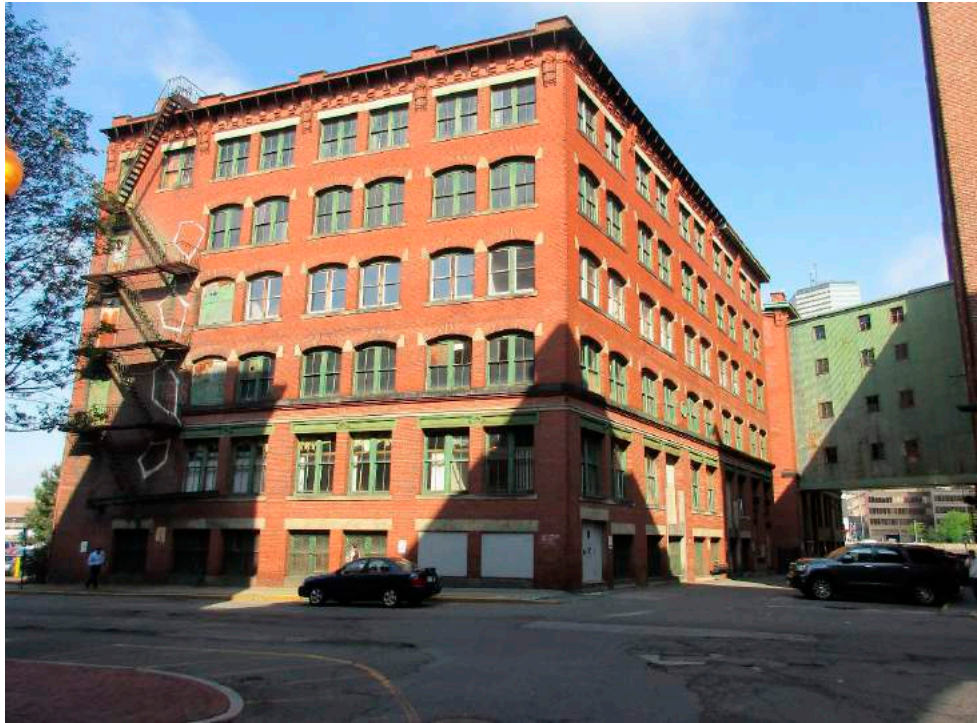
1. View west of 5 Necco Court from intersection of Necco Court and Necco Street
