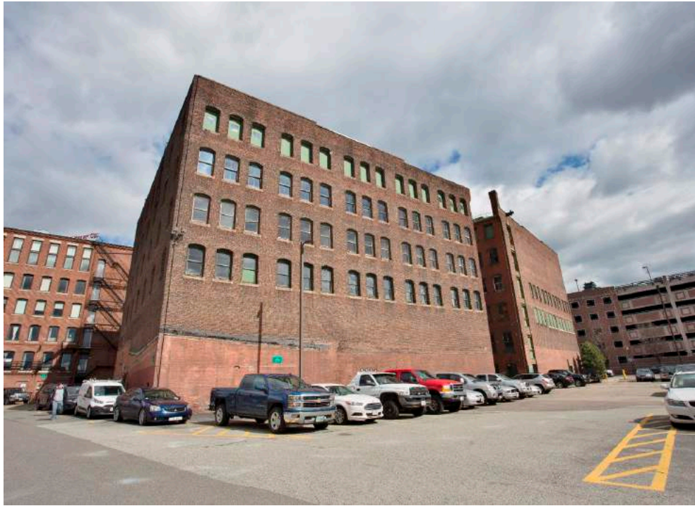
5. View northeast of 5 and 6 Necco Court from east bank of Fort Point Channel
