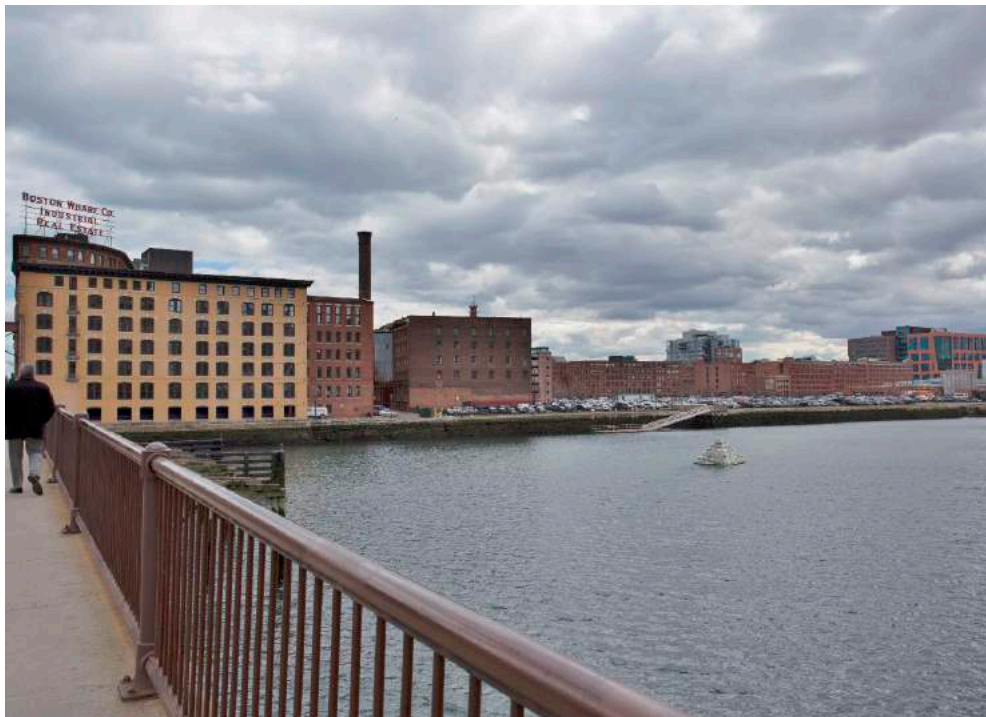
18. View southeast towards 5 and 6 Necco Court from Summer Street Bridge
