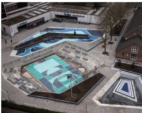
Figure 160. Multi-use detention basin, Rotterdam, Netherlands
