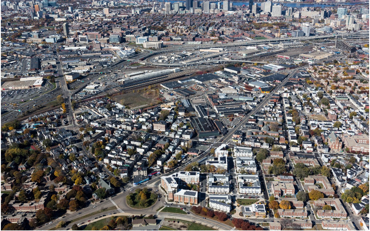
Figure 88. Aerial image of the district
