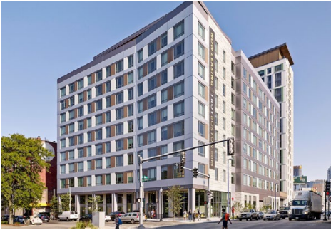
Figure 173. The structured parking is wrapped with residences and an active ground floor, Troy Apartments, Boston
