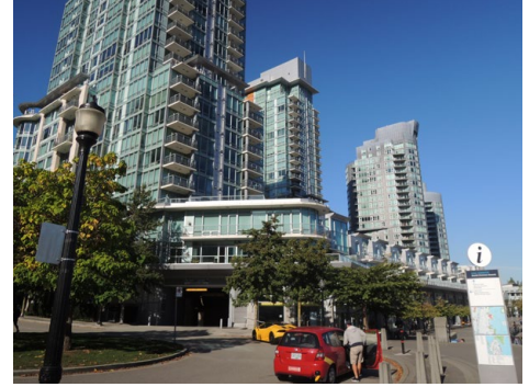
Figure 169. A series of towers are linked by a common podium that is active in use along the main pedestrian thoroughfare, Vancouver, BC.
