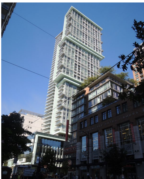
Figure 164. The tower is set back from the primary street wall and is closer to the side street, Vancouver, BC.
