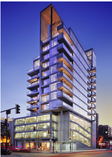
Figure 174. The podium garage is clad in high quality glazing that matches the tower above, Contemporaine, Chicago
