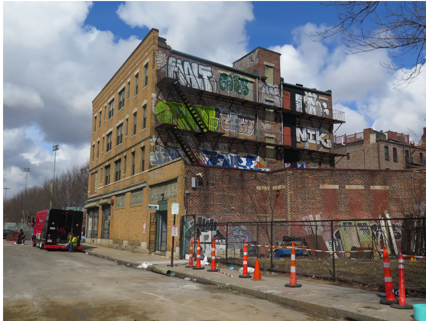
View of Rear of 1938-1946 Washington St from Thorndike St
