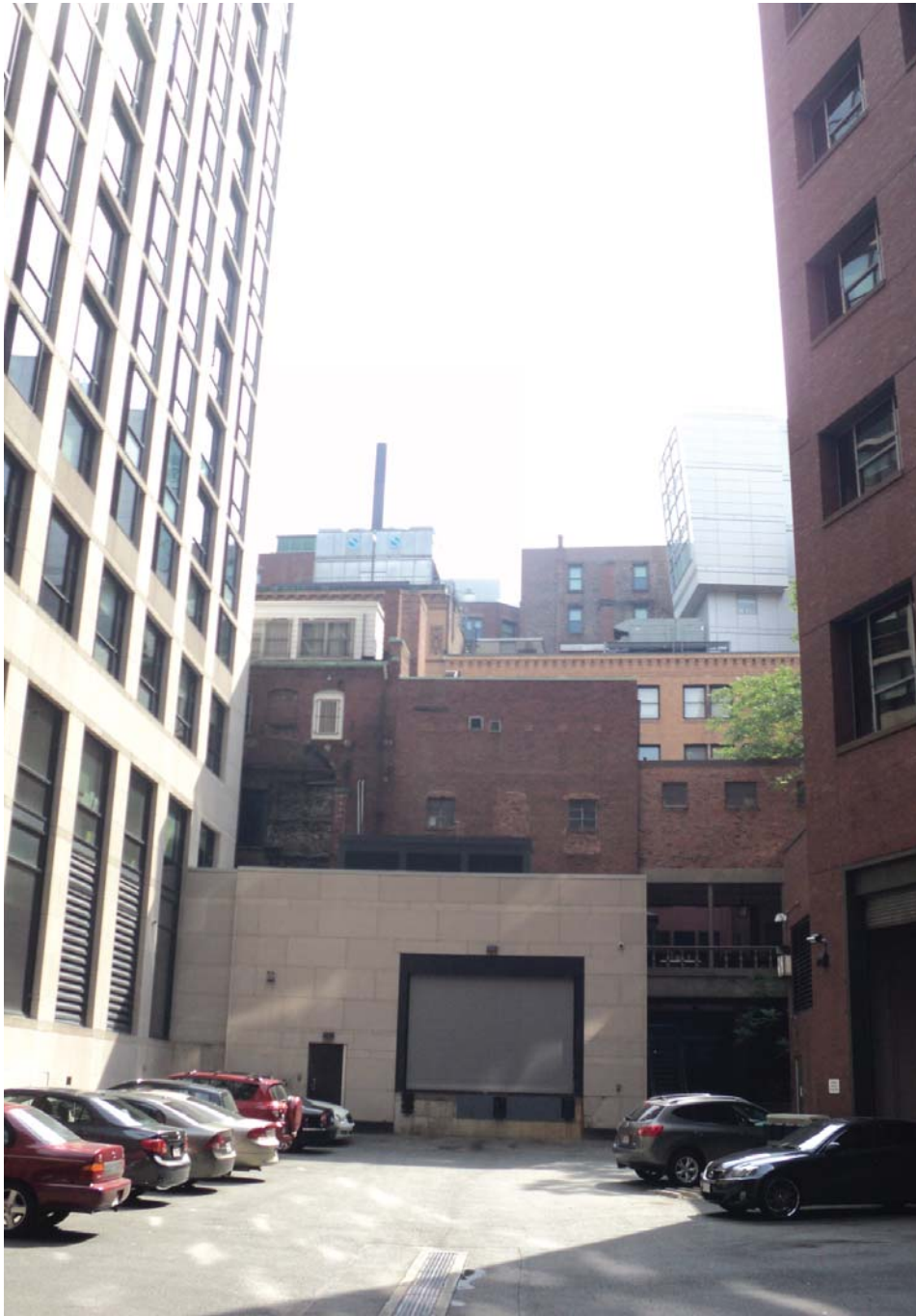
View East, Piano Row Residence Hall loading dock
