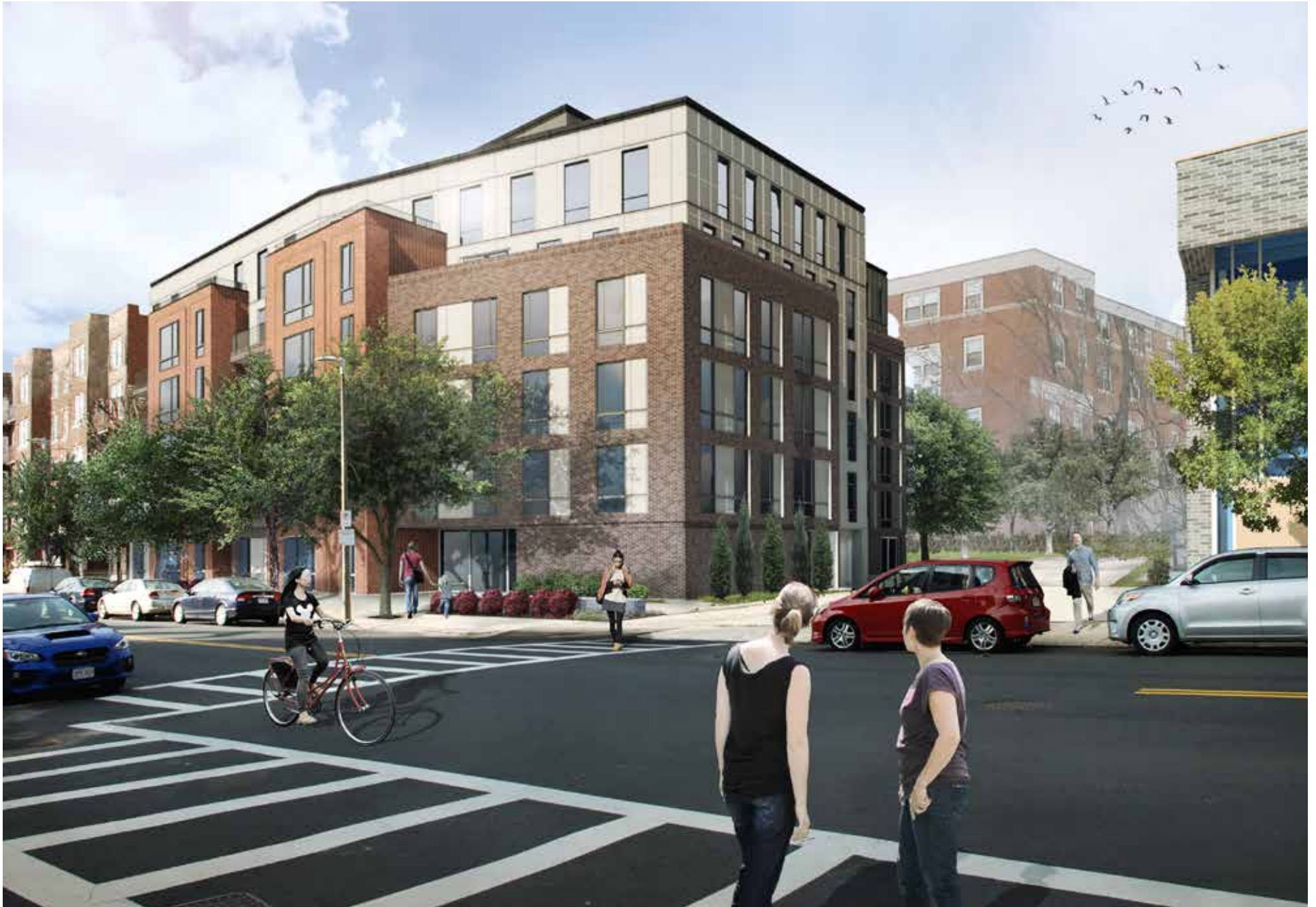
View of 105 Washington from across Washington Street
