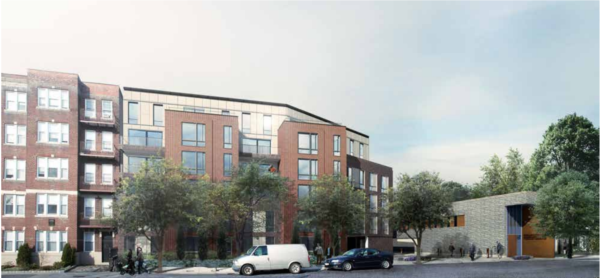
View of 105 Washington from across Washington Street
