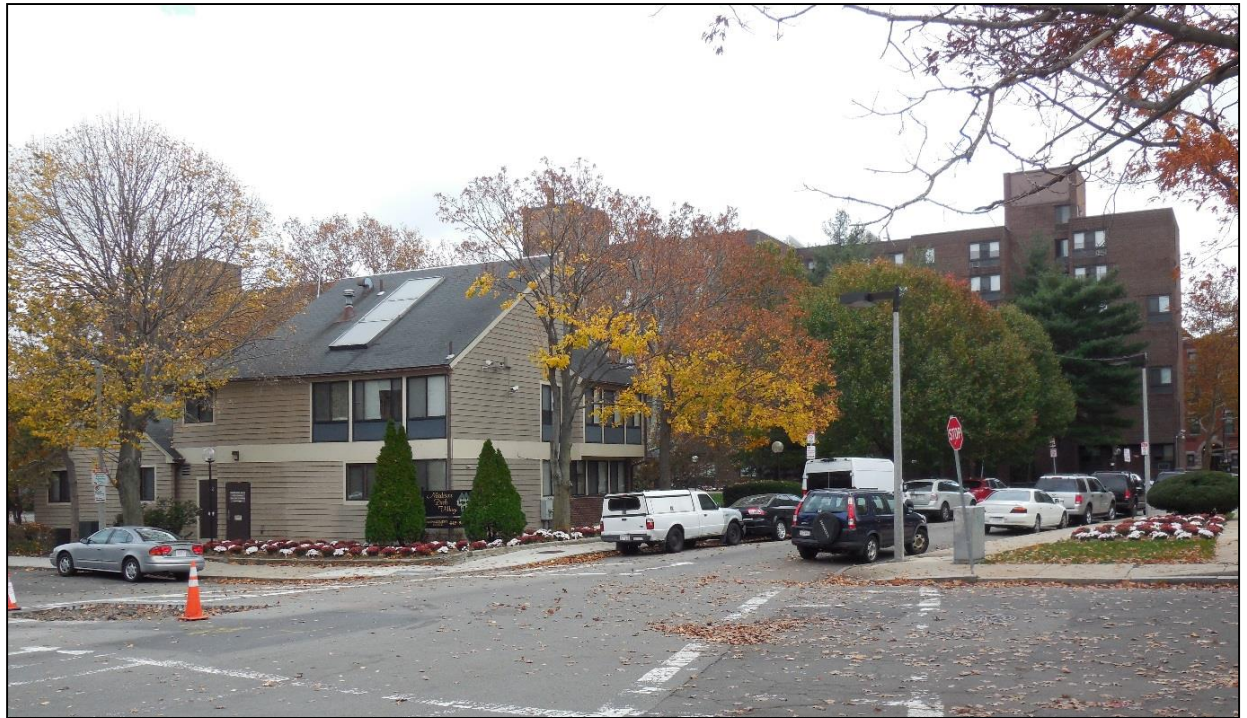
Figure 6 - Existing Conditions – View of Site from Dewitt/Ruggles Intersection
