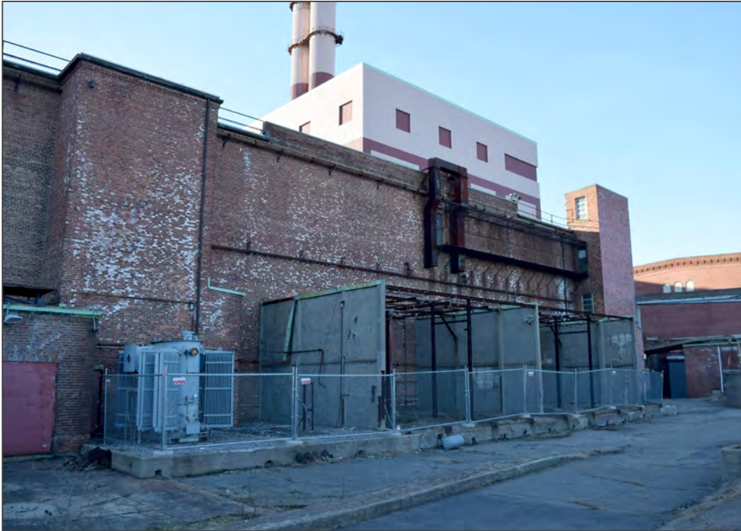
21. Facing west toward east elevation
