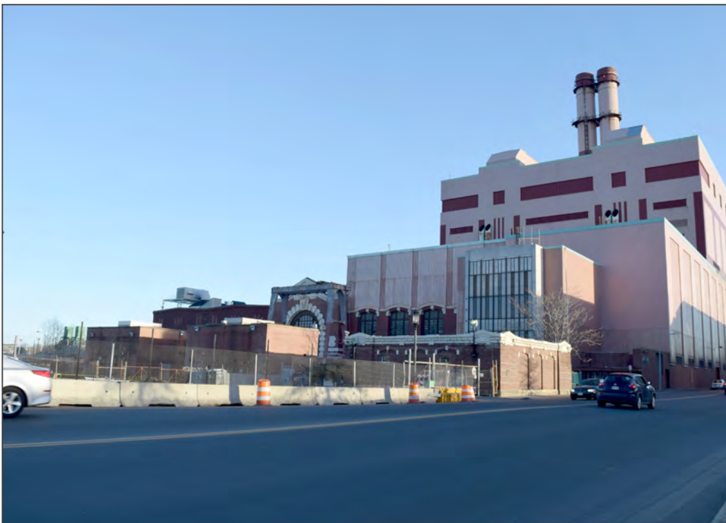
36. Facing south toward north elevation
