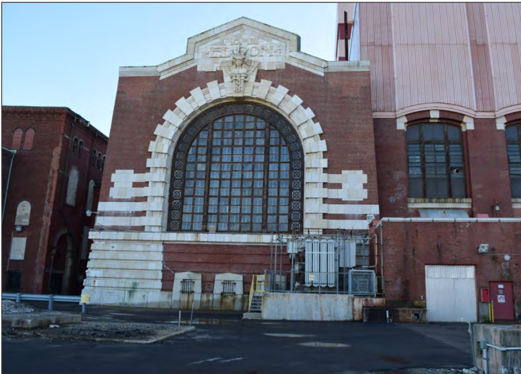
4. Facing south toward north elevation
