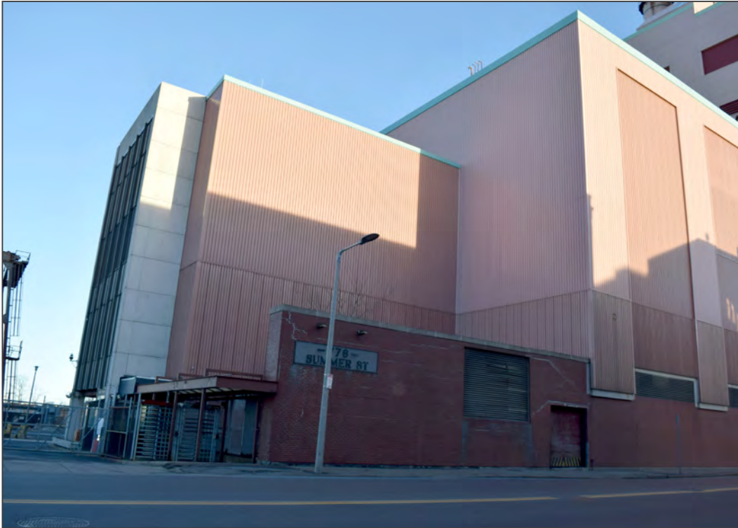
35. Facing southeast toward north and west elevation
