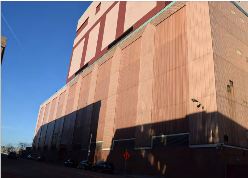
34. Facing northeast toward west elevation
