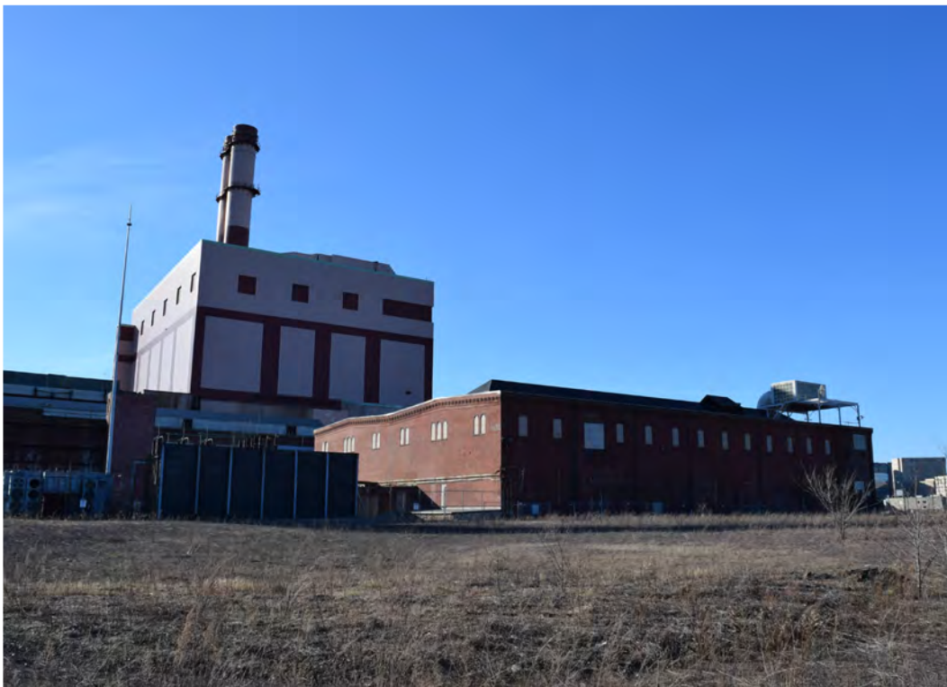
14. Facing northwest toward east elevation
