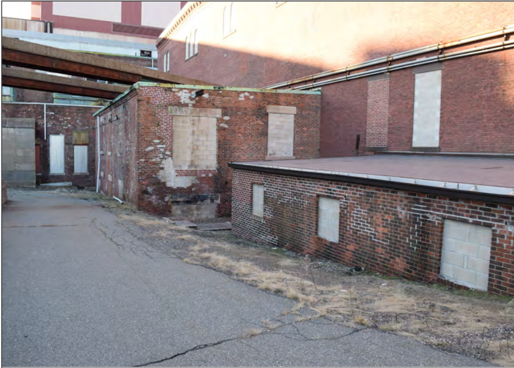
15. Facing northwest toward east elevation
