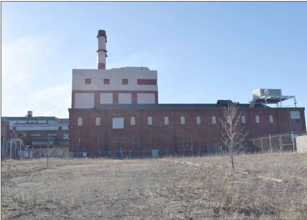
12. Facing west toward east elevation
