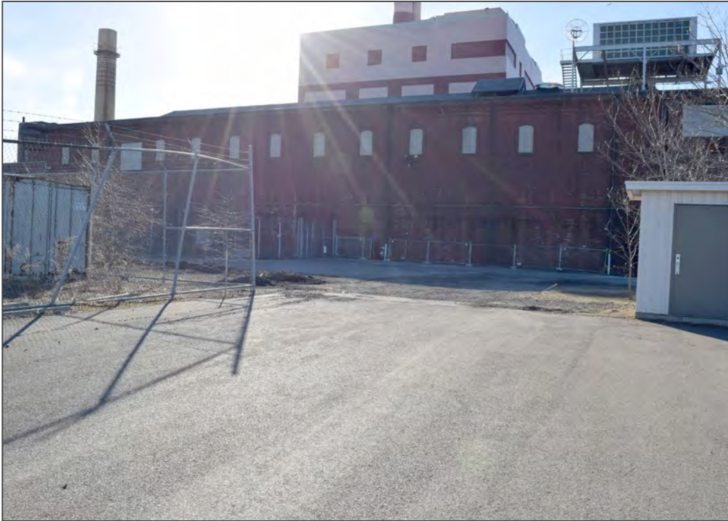
11. Facing west toward east elevation
