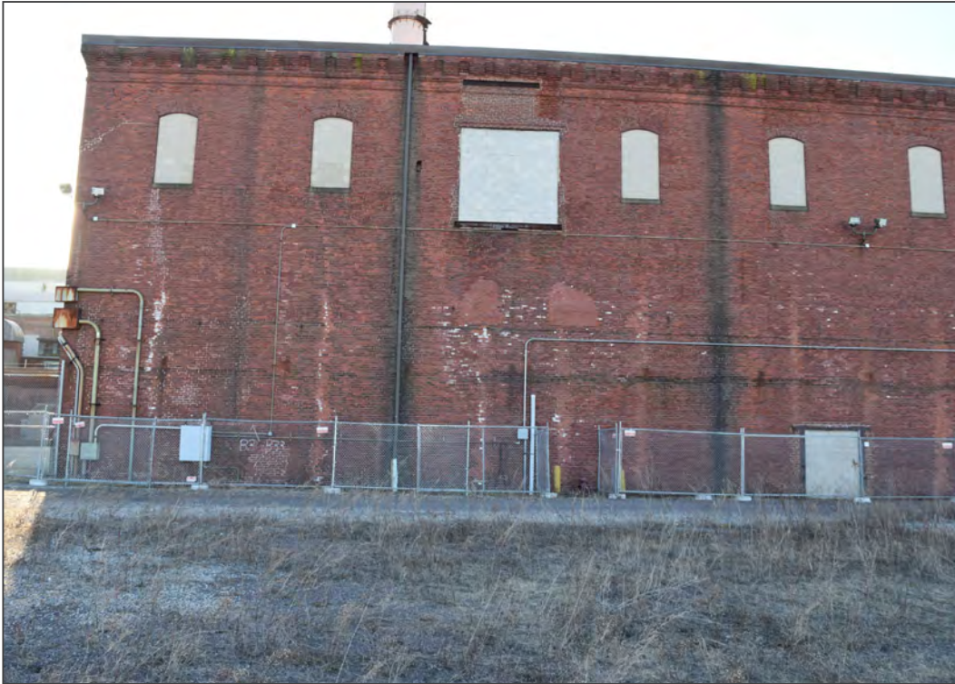
13. Facing west toward east elevation
