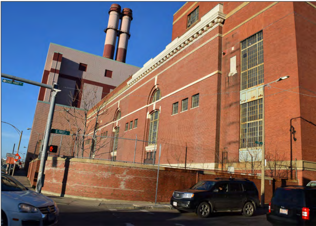
28. Facing northeast toward west elevation
