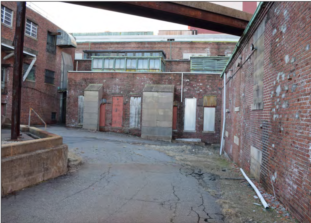
16. Facing west toward east elevation
