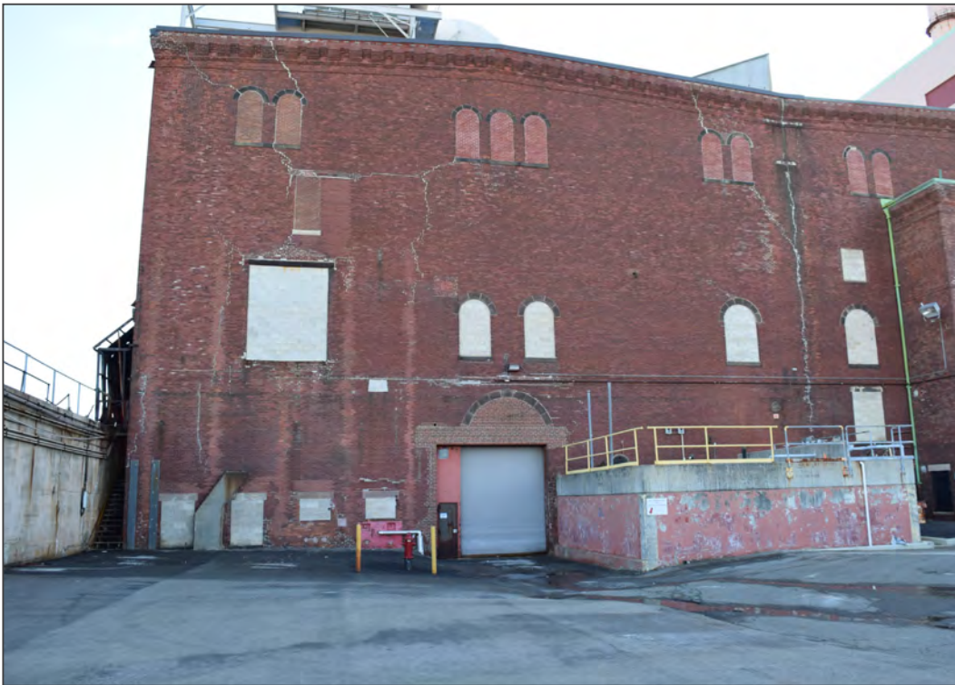
8. Facing south toward north elevation
