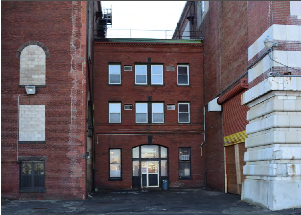
5. Facing south toward north elevation
