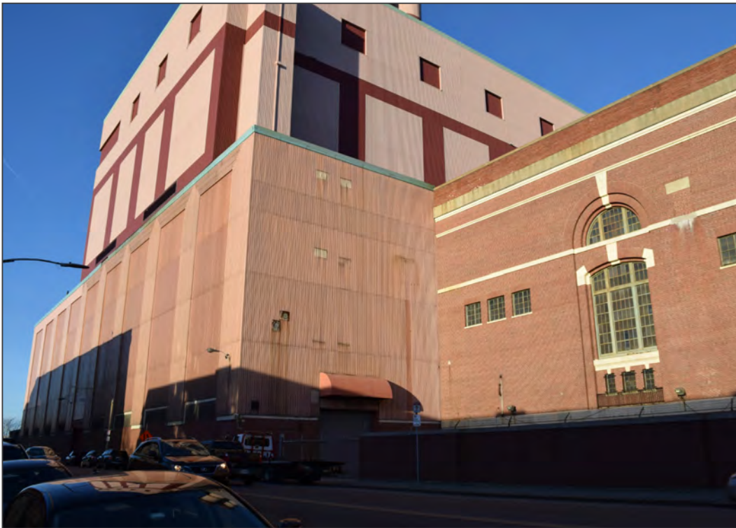
32. Facing northeast toward west elevation
