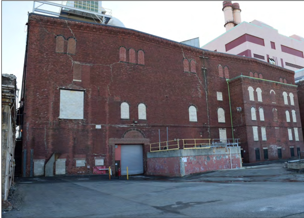
9. Facing south toward north elevation
