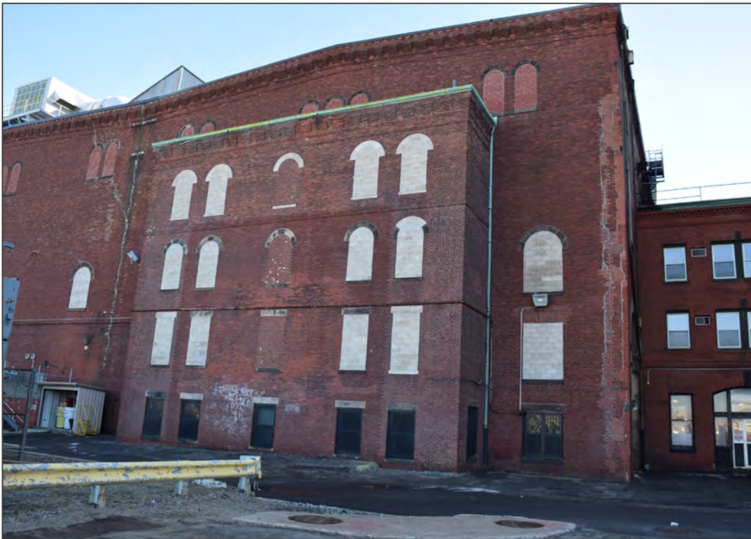
6. Facing south toward north elevation
