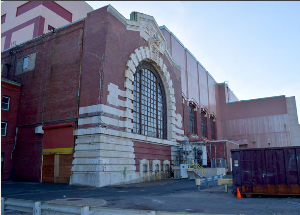
7. Facing southwest toward north elevation
