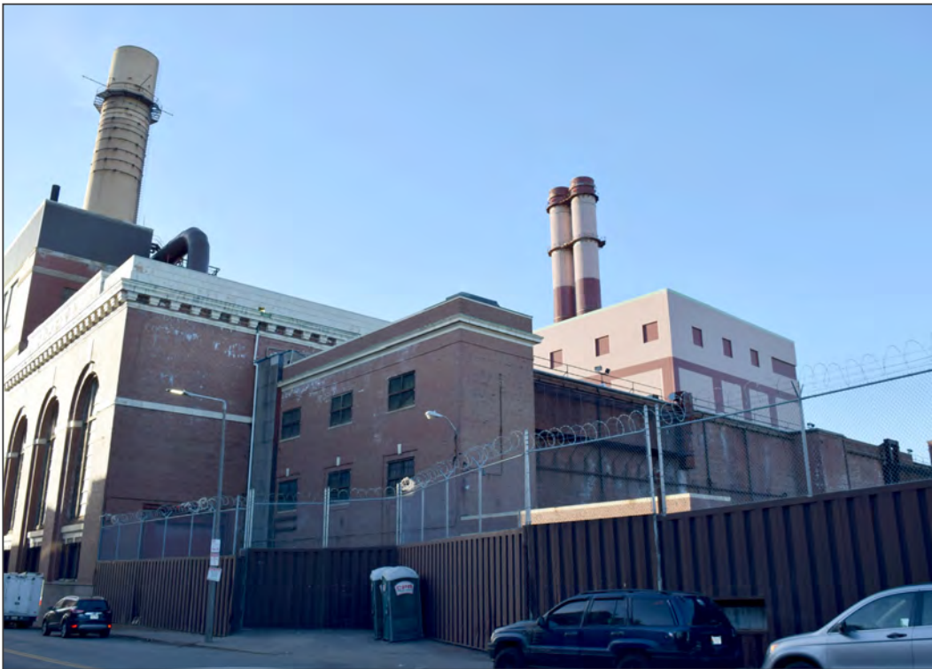
24. Facing northwest toward east elevation
