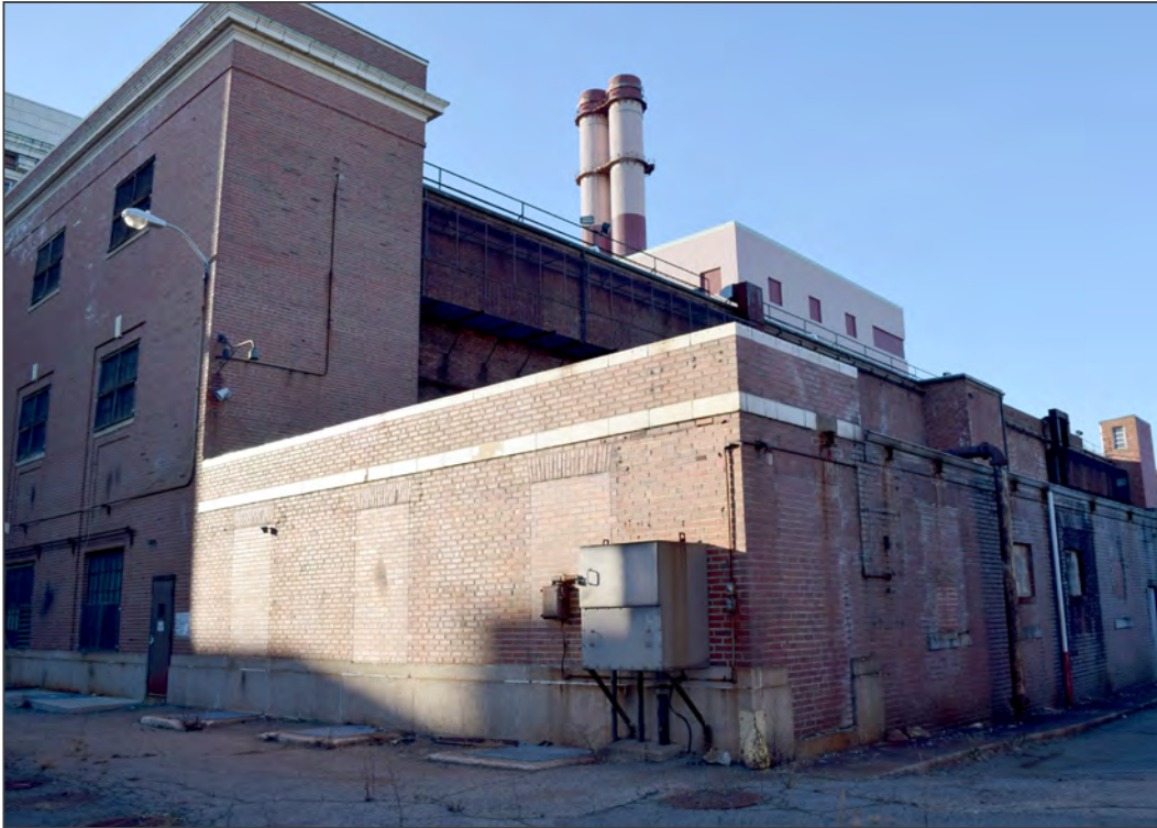
23. Facing northwest toward south and east elevations
