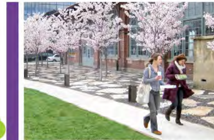
RECYCLED CONCRETE SLABS Navy Yard, Philadelphia
