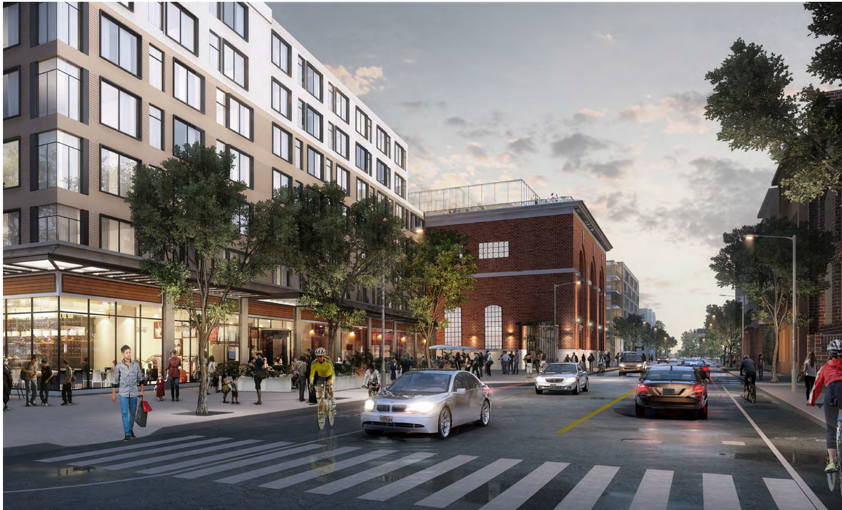
L Street Station Redevelopment | Boston, Massachusetts
