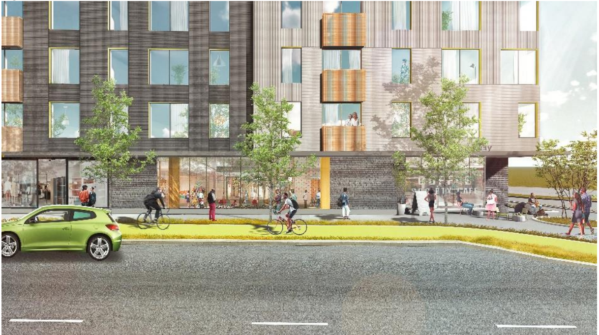
Figure 2-28: River Street Facade
