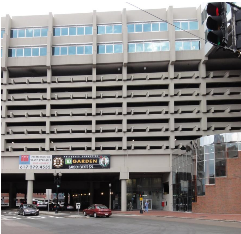
View from Merrimac Street
