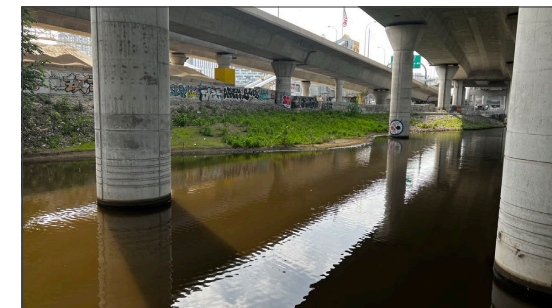
Stormwater and groundwater pollutants are mitigated before they reach the existing sediment-impacted Millers River, helping to improve water quality and ecological capacity.
