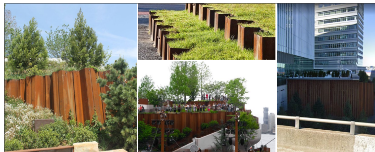
Steel piles on either side of 6 foot wide planting beds raise phytoremediation trees 10 to 20 feet into the air, helping to mitigate air pollution from the elevated Interstate 93 highway.
