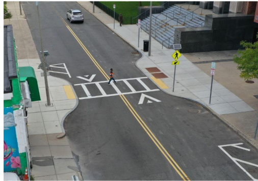
A raised crosswalk in Roxbury.
