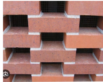
Full Depth Modular Brick Screen_ Parking Walls
