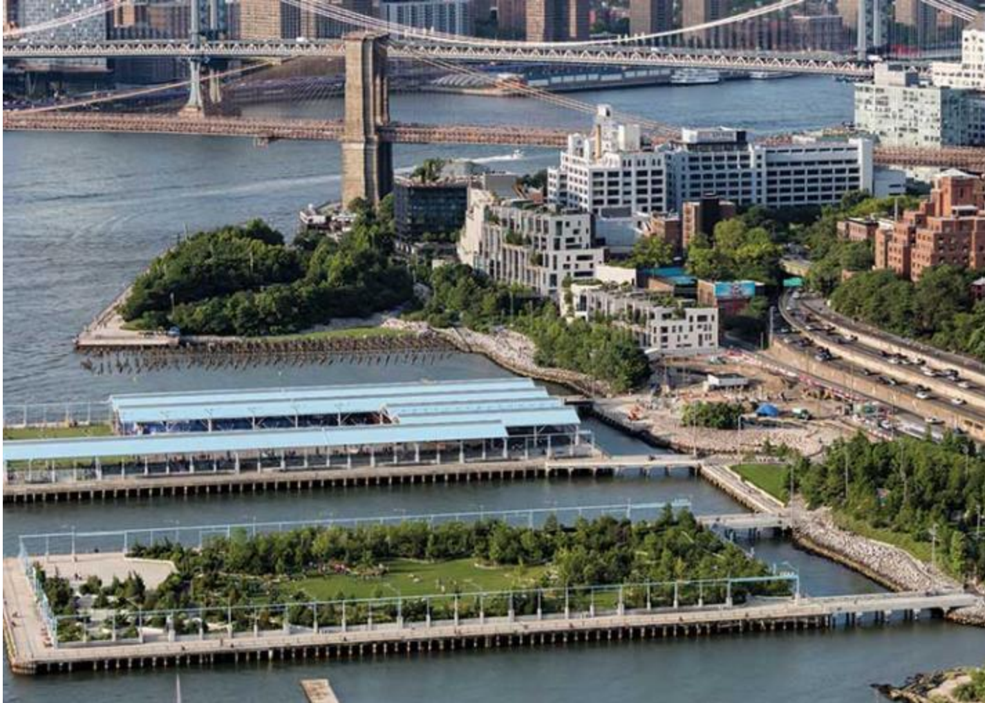
Brooklyn Bridge Park, NY
