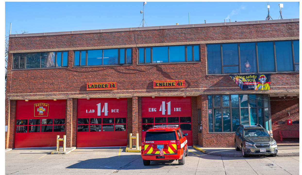
Photo of Boston Fire Department Engine Company 41 and Ladder 14
