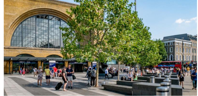
Transit Gateway (Kings Cross Station, London, UK)
