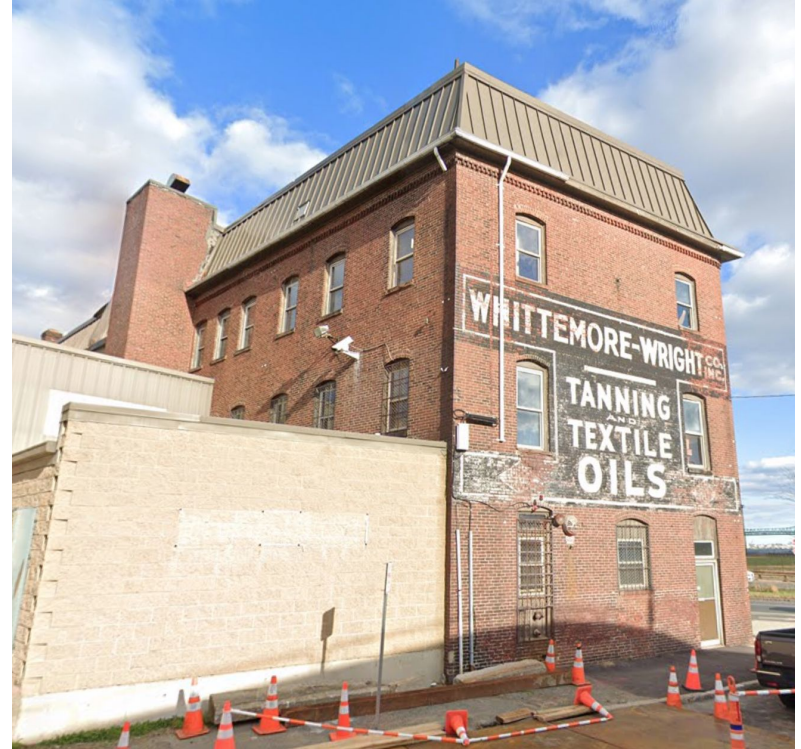
Whittemore- Wright Tannery Building, 62-68 Alford Street, Charlestown
