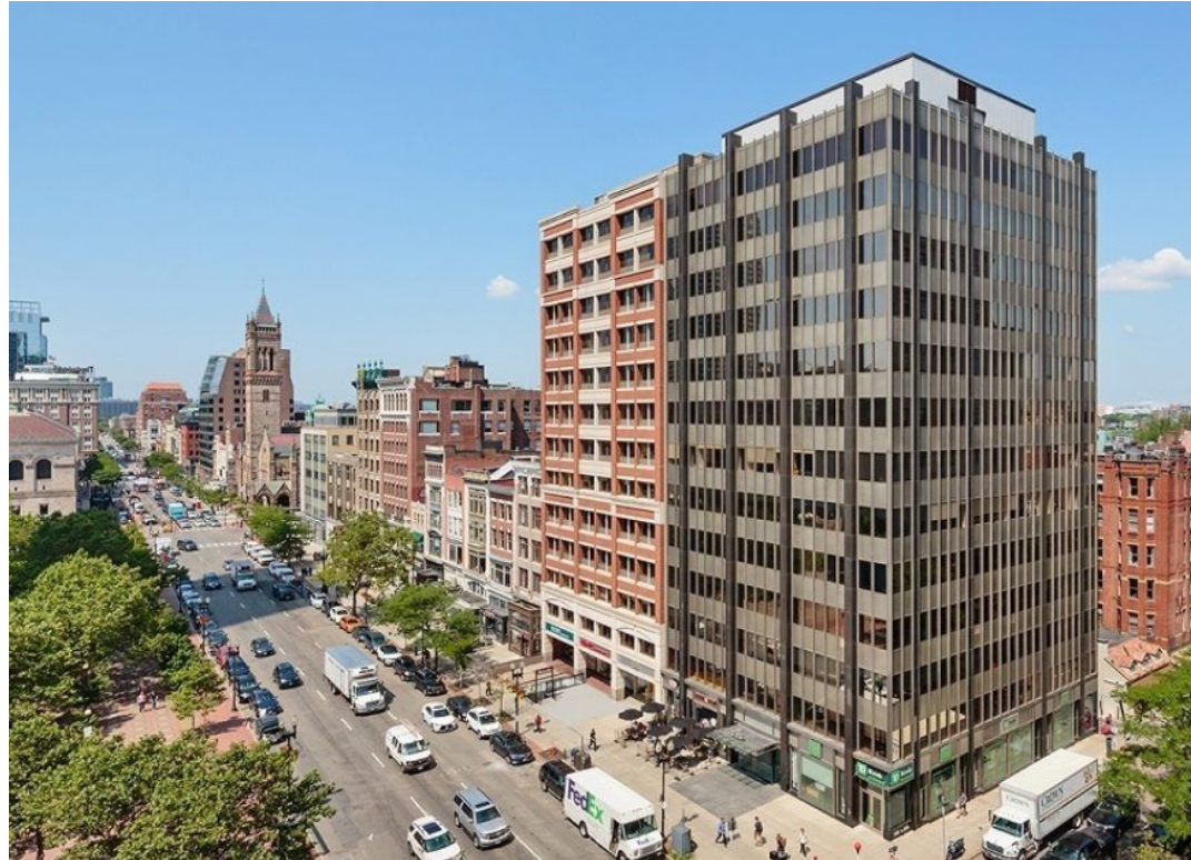
535-545 Boylston - Partial conversion of office floors to lab space
