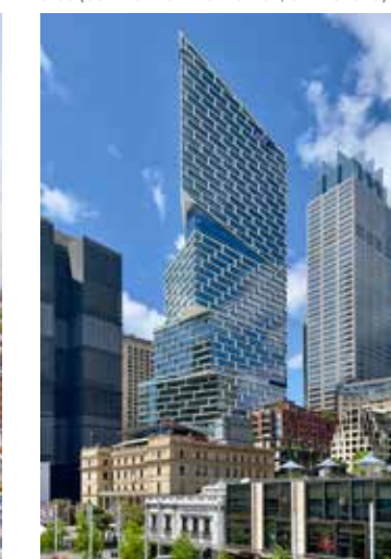
Quay Quarter Tower reuses an existing 1976 tower reaching the end of its usable lifespan to create a more sustainable tiered massing. (3XN, Australia)
