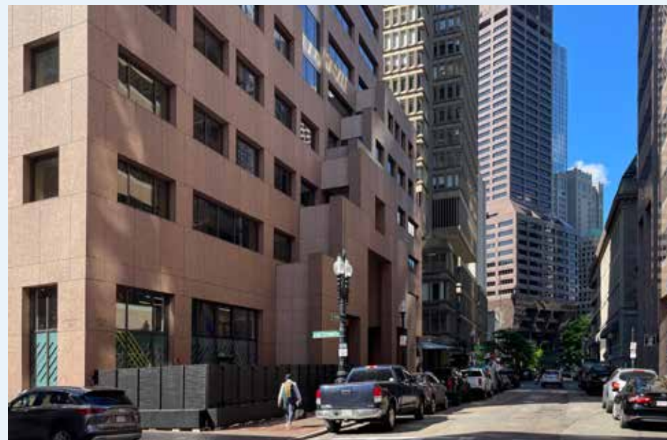
Large-scale commercial buildings in the Financial District
