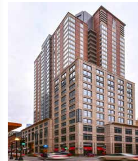
660 Washington stepbacks at a height aligned with neighboring historic buildings. A higher stepback at the corner helps break up the massing and emphasize the tower corner. (Boston)
