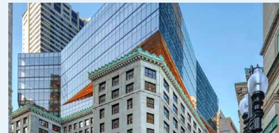
The Congress Square project by Arrowstreet in 2015 adaptively reused existing historic buildings, restored existing facades, and added a modern addition above the existing historic structures.
