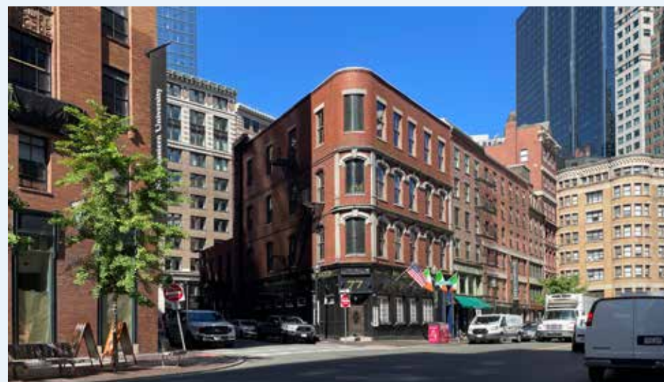
Cohesive scale of warehouse buildings along Broad Street
