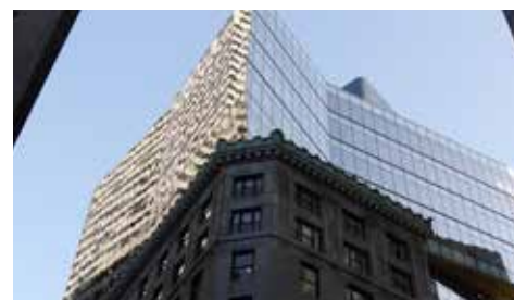
Setback cornice - Boston, USA
