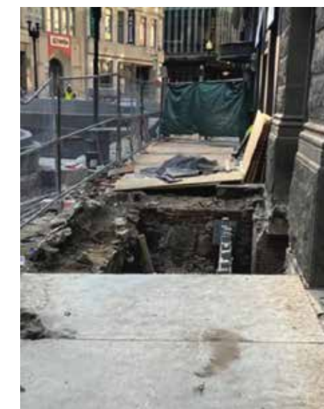
An areaway uncovered on Franklin St
