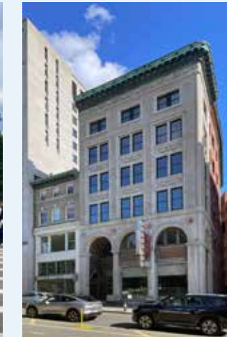
The Steinert Building (1896)
