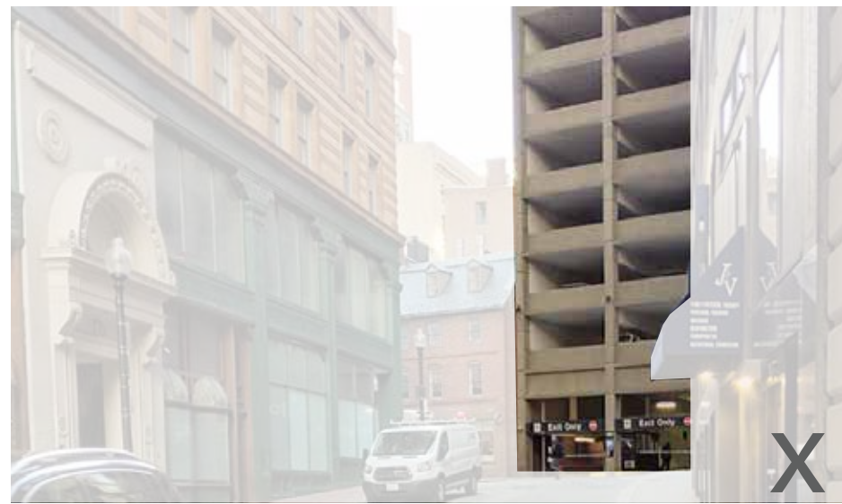
View to structured parking at end of Water Street
