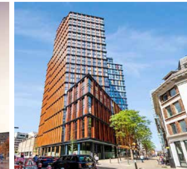
One Crown Place Towers' facade is distinct from neighboring buildings, but tiered stepbacks help transition tall portions of the tower to the lower historic context. (KPF, Canada).
