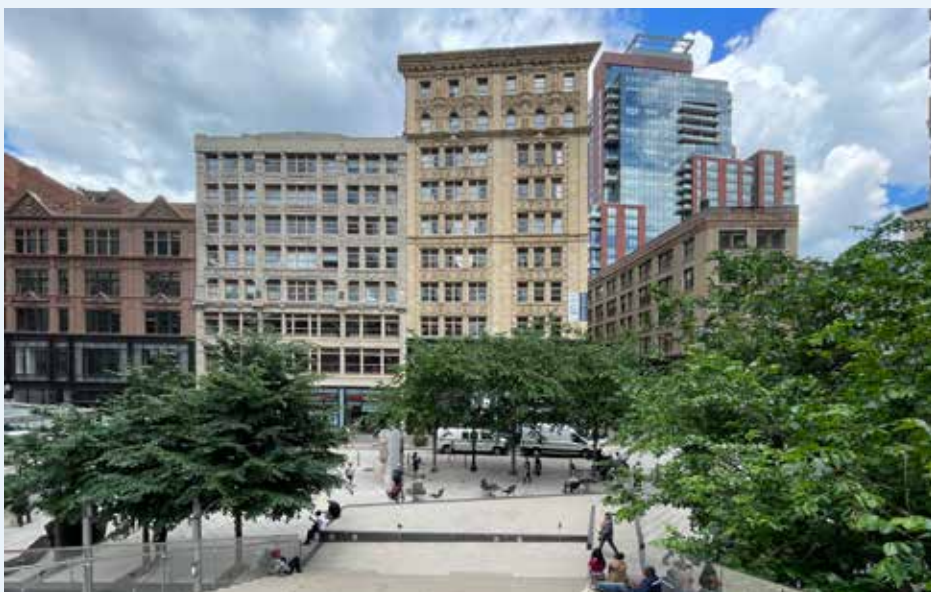
Historic street wall along Washington Street; view from the Shopper's Plaza amphitheater Right: Contemporary public space at Tontine Crescent, with curved street wall
