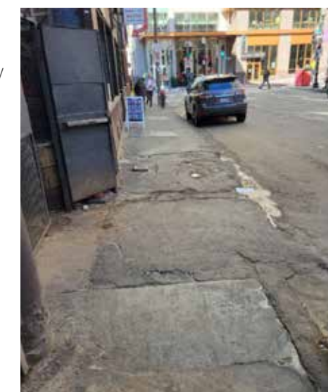
Sidewalk in Chinatown with areaways underneath
