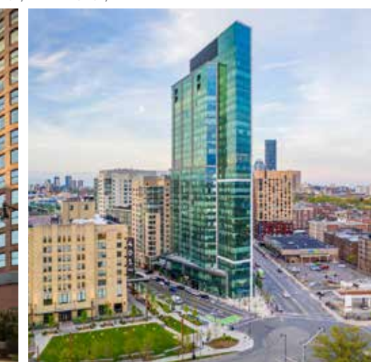
The 188 Brookline Ave residential building's front corner setback makes a small public plaza. Small podium-level stepbacks along each side of the tower help mitigate negative height impacts on the street. (CBT, Boston).
