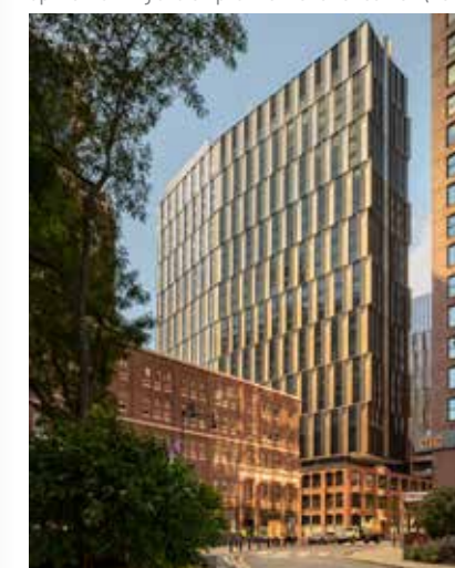
Site 4 graduate housing reuses a brick warehouse building and orients the primary massing away from the street edge. (NADAA, Cambridge)
