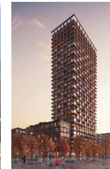
Rocket & Tigerli mass timber tower design uses terracotta brick to complement the surrounding area (Schmidt Hammer Lassen, Switzerland)
