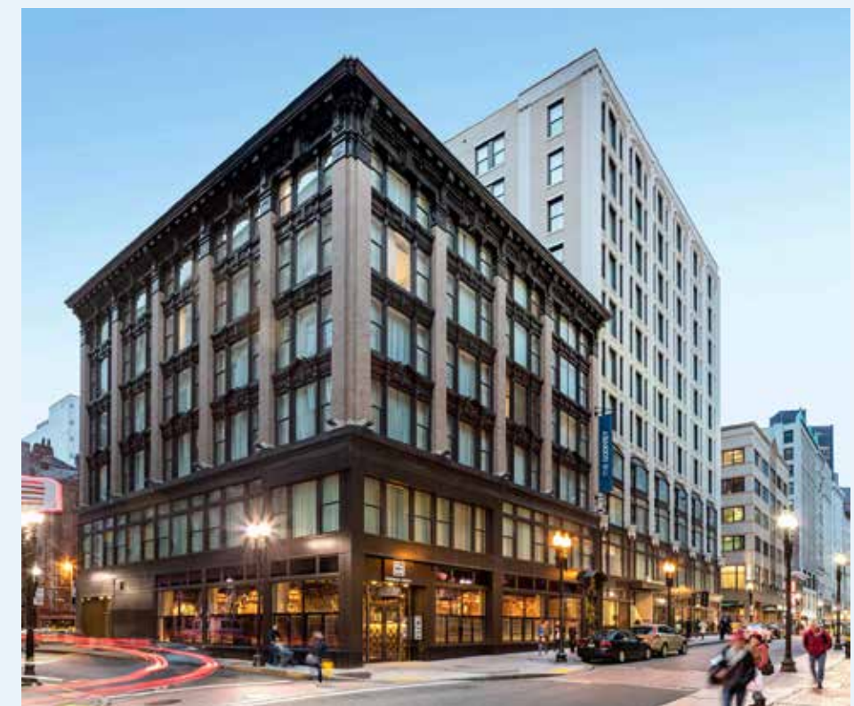
Godfrey Hotel conversion of vacant office buildings to hotel and ground floor retail.
