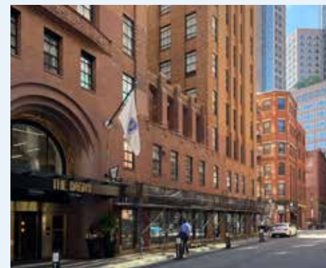
Relationship of the Batterymarch Building facade (1918) to the frontage of Broad Street
