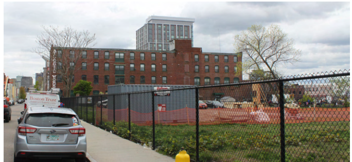
FIG 03-24 VACANT LOT AT 102 BORDER STREET. [TOP]
