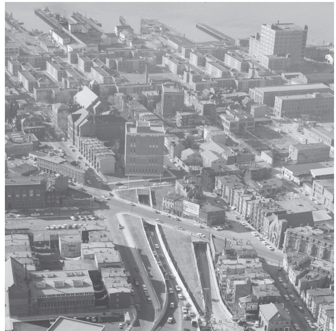
FIG 01-20 AERIAL IMAGE OF THE CALLAHAN AND SUMNER TUNNELS (C. 1955-1964)
