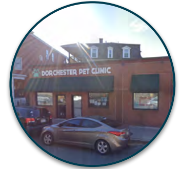
Some small offices on the ground floor
