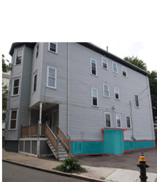
Basement conversion - convert basement into an accessible unit
