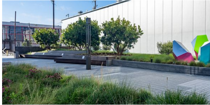
The Manufacturing Foundry, - Light manufacturing building in San Francisco
