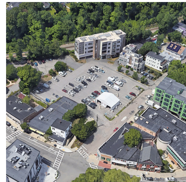
Aerial: Taft Hill Municipal Parking Lot
