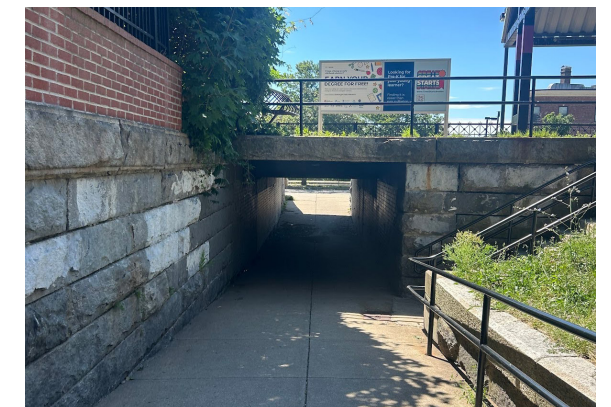
Pedestrian Underpass at MBTA Commuter Rail Station
