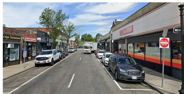
Tight fabric of small-scale one- and two-story commercial storefronts along Corinth Street, Poplar Street, and South Street
