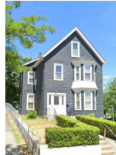
Example of a gabled roof
