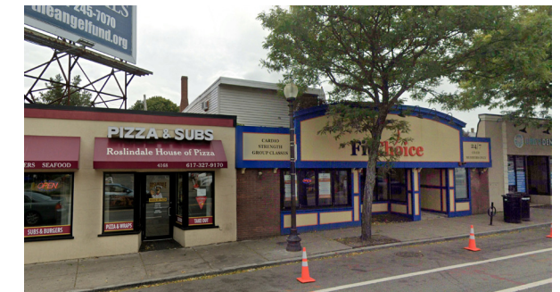
One- and two-story commercial storefronts on the southeast side of Washington Street
