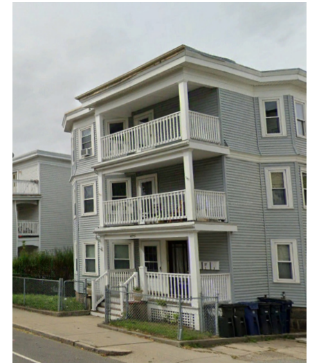
Example of a flat roof
