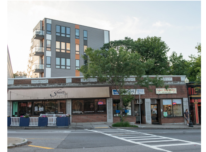
Residential and Commercial along Washington St
