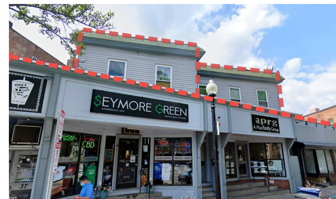
Upper story setbacks on the second floor of a Poplar Street storefront
