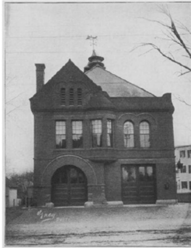
ROSLINDALE FIRE HOUSE
