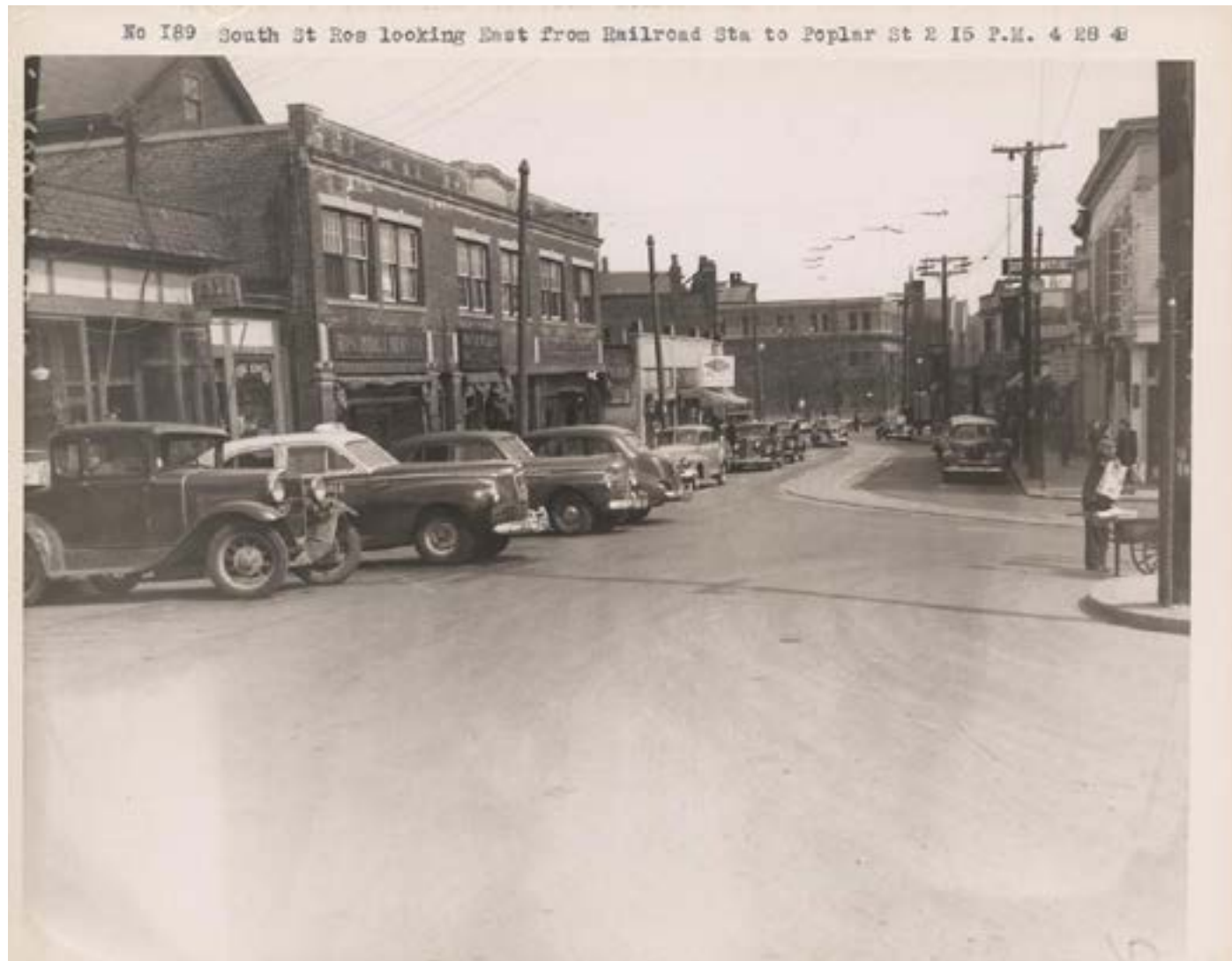
Figure 9. View along South Street, 1948. Note historical architectural details which reference previous popular architectural trends. Features that may be associated with one or more of these various “Revival” styles include columns flanking doors and windows; keystones at the center of the lintels above the windows (center left); orderly facades framed by cornices above shop windows and at the roofline; and the use of wood and stucco mimicking medieval half-timber construction. Boston City Archives.
