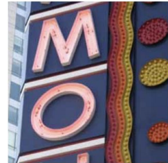
Channel Neon Tube Light is emitted by neon tubes mounted inside channels, creating a glow effect.
