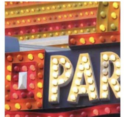
Exposed Incandescent Exposed bulbs mounted to the face of a sign create the illumination.
