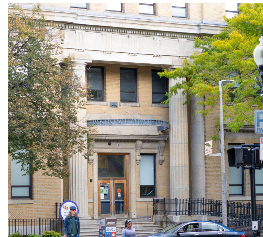
Roslindale Community Center
