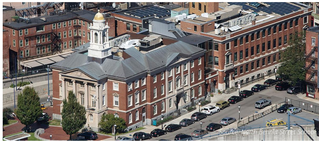
North Bennet Street Trade School, North End
