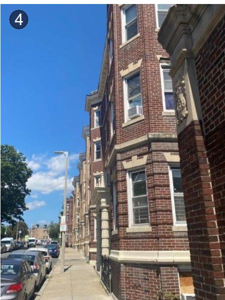
4 View toward FC from Comm. Ave. Residential 4+ Story
