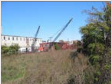
Carlton Wharf site - before
