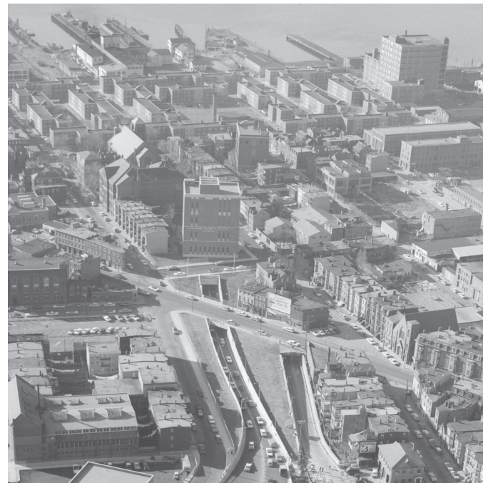
FIG 01-13 AERIAL IMAGE OF THE CALLAHAN AND SUMNER TUNNELS (C. 1955-1964) Construction of the Sumner Tunnel (opened in 1934) and Callahan Tunnel (opened in 1961) cut through the middle of the area and required the demolition of established residential fabric between Liverpool Street and Havre Street. Today ventilation facilities for both tunnels loom large over residential buildings in the area. Image accessed via Northeastern University Library, Archives and Special Collections.
