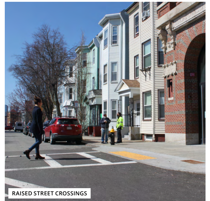
FIG 01-10 EXAMPLE STREET SAFETY AND GREEN INFRASTRUCTURE TOOLS (Clockwise from top left) Curb extensions with bioretention, clear corners, street trees with porous pavers, raised side street crossings, and speed humps Source: Boston Streets Cabinet
