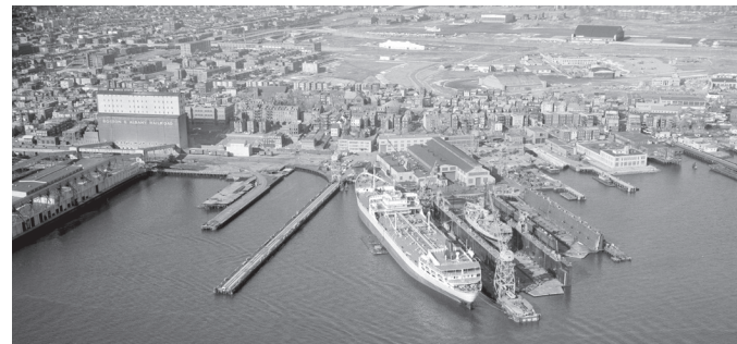
FIG 03-14 MARGINAL STREET WATERFRONT (CA 1955 - 1964). Industrial facilities pictured here include Bethlehem Steel Company, now the Boston Harbor Shipyard & Marina, and the Grand Junction Railroad and Wharves, now open space associated with Piers Park. Image accessed via Northeastern University Library, Archives and Special Collections
