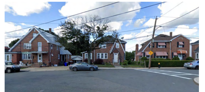
FIG 01-61 While much of Orient Heights contains small, one-to-two story buildings, larger buildings are not uncommon throughout the area, especially closer to Bennington Street and Orient Heights square. Large development proposals in the adjacent industrial and economic development areas will create additional density nearby. It is important for new zoning to mediate between these conditions and create an appropriate transition between different scales of development.
