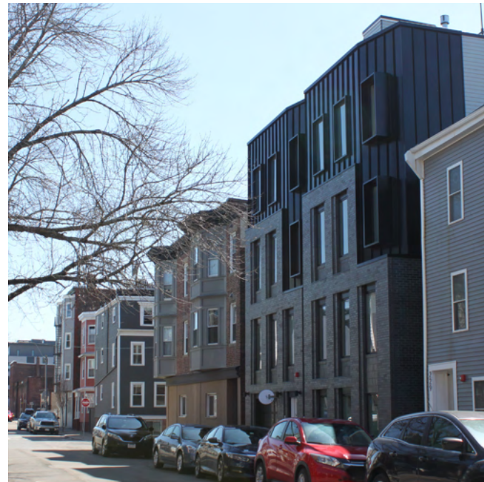
FIG 01-38 231 MAVERICK STREET (2023) Example of infill development along Maverick Street.
