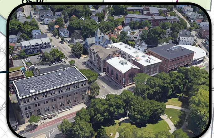
Wide buildings that cover most of the lot and hold active and housing uses
