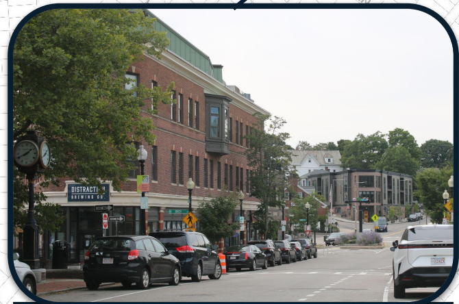
Existing mixed-use and multi-story multiple buildings with commercial spaces on the ground floor
