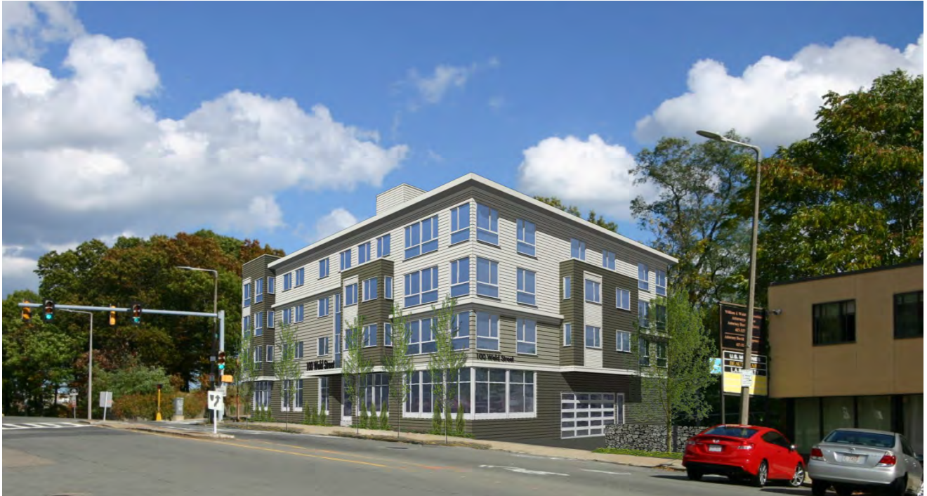
View of Centre Street façade looking north
