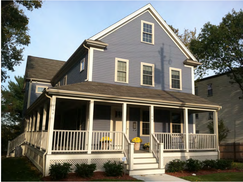
194 - 196 Durnell Avenue, Roslindale ... 2-units, new construction
