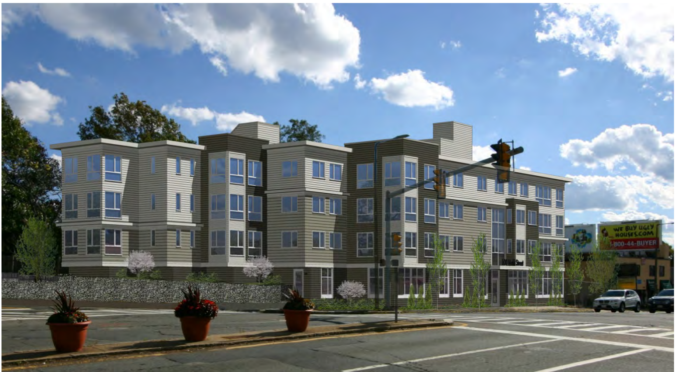
Corner view of Weld and Centre Streets façades looking south
