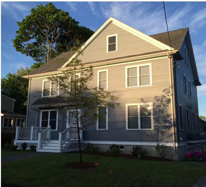
Warren Avenue, Hyde Park ... single-family, new construction.
