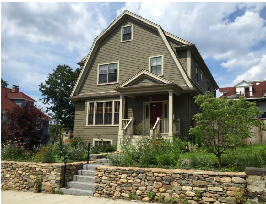
17 Park Lane, Jamaica Plain ... single-family, new construction
