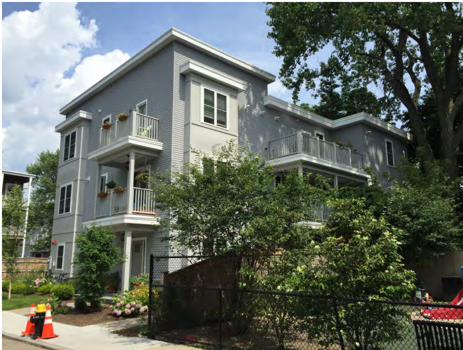
8 - 12 Stedman Street, Jamaica Plain ... 3-units, new construction
