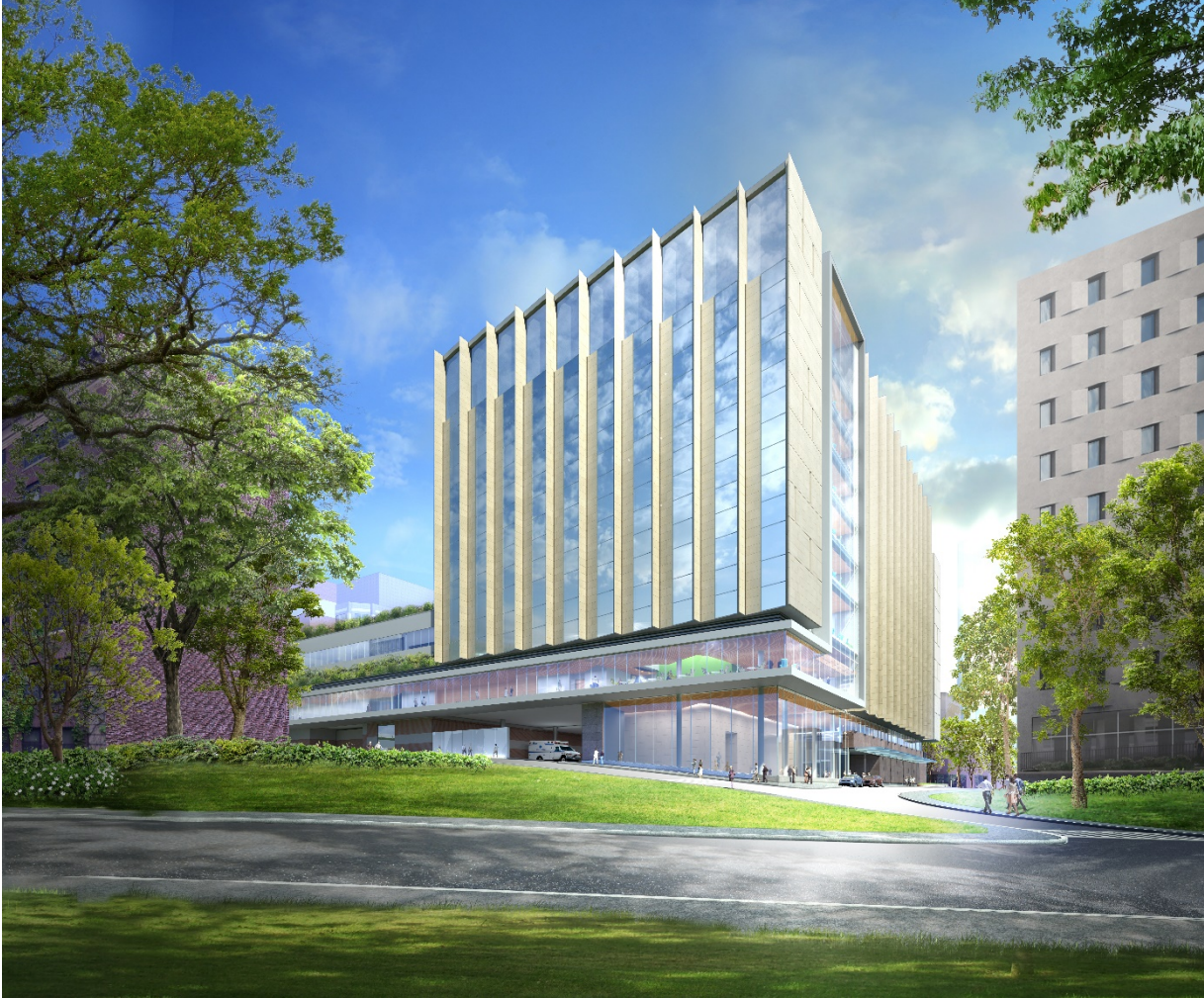
PALMER BUILDING IN FOREGROUND REMOVED FOR CLARITY
