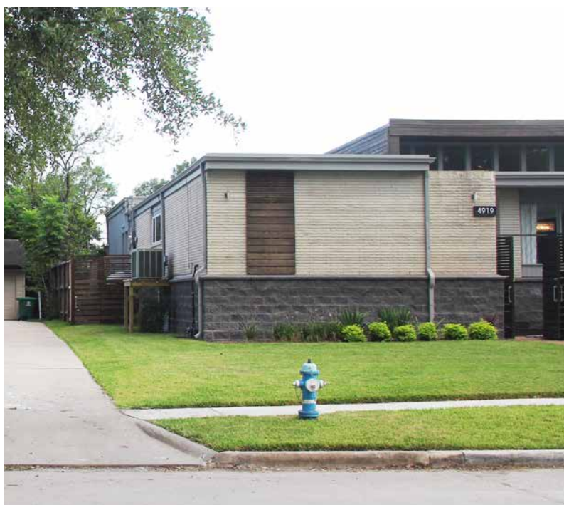
House after elevating. Note that the condenser is also elevated at left. Flood vents are not pictured.
