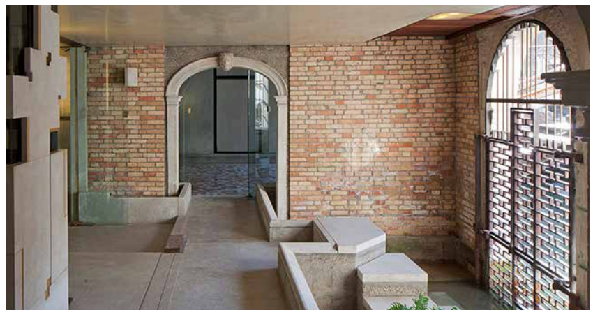
Floodable entryway with stairs that lead to an elevated lobby at the Querini Stampalia in Venice, Italy. Photo: Architectours / "The renovation of the Fondazione Querini Stampalia is a great example of how Master Carlo Scarpa integrated the new with the old"
