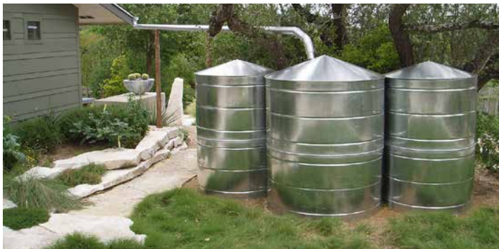
Photo: Innovative Water Solutions LLC / "Galvanized Metal Cisterns"
