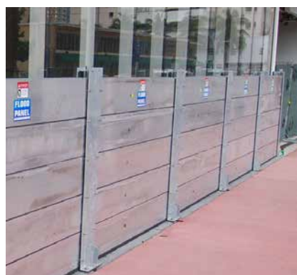
Drop-in flood shields inserted into brackets Photo: Flood Panels LLC
