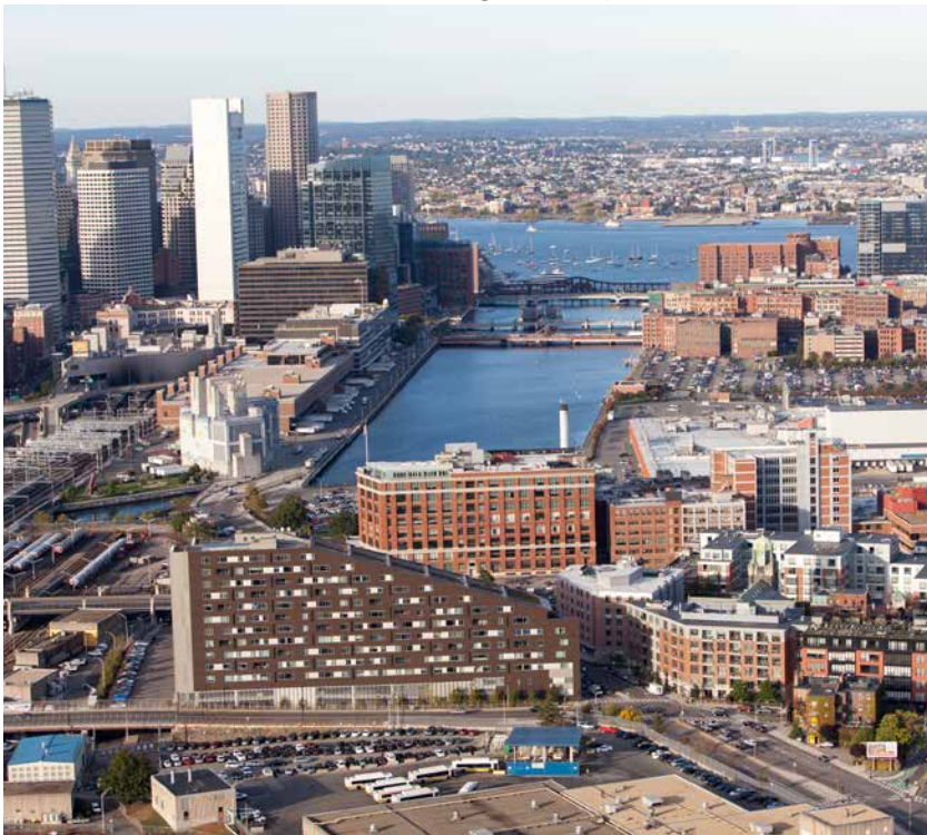
The Fort Point Channel is a major inundation point for the 1 percent annual chance flood risk in the year 2070. Photo: Landslides Aerial Photography / Alex MacLean
