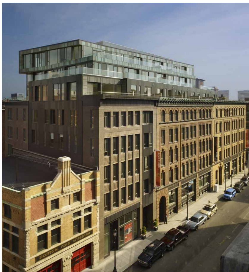
Rooftop addition to an existing pre-war mixed-use building in the Fort Point neighborhood. Source: Hacin and Associates / FP3
