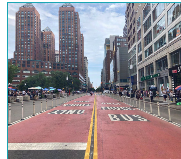
14th Street Busway in New York City
