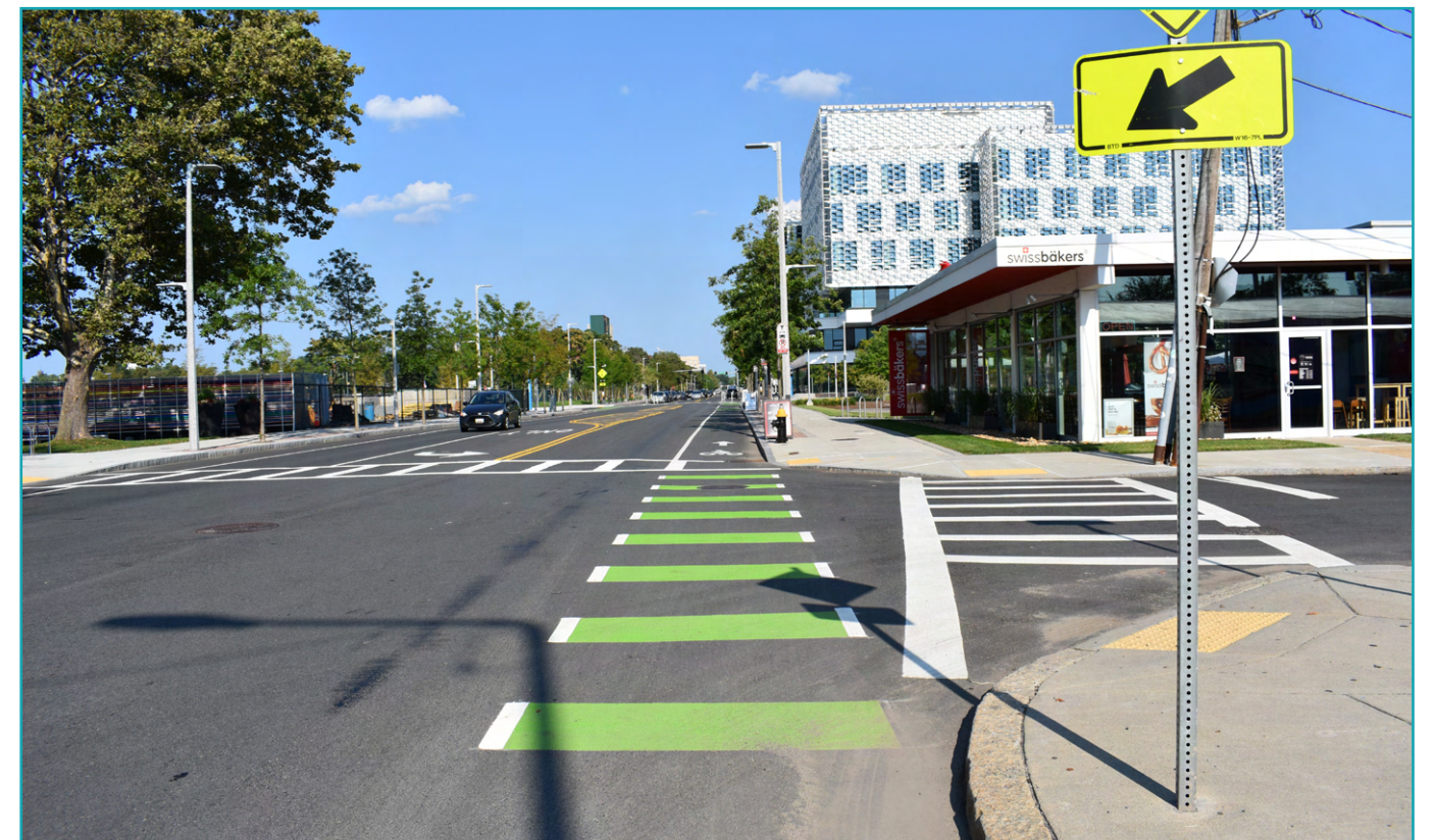
Bike Infrastructure on Western Avenue today, leaving the study area. This bike lane is clearly delineated with a high visibility conflict area.
