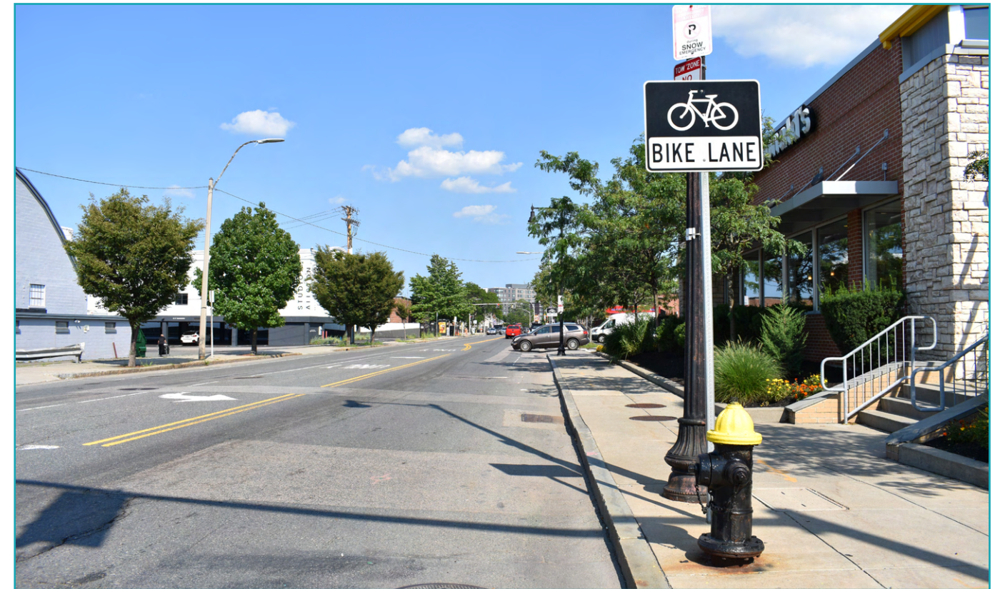
Bike Infrastructure on Western Avenue today. Bike lanes are marked with signage, but space is not marked or designated on the roadway itself.
