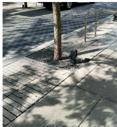
Shopper's Plaza pavement
